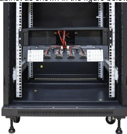
Fig. 3. The battery mounting method.
